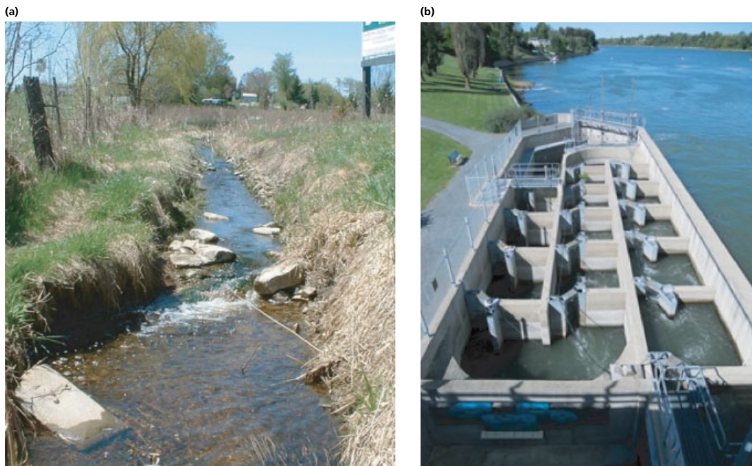
Figure 6.3.5 (a) Small nature-like fishway to facilitate passage at a low-head dam and (b) a constructed vertical slot fishway at a barrier on a large river.
